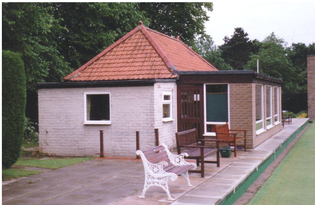
Pavilion Extension, 1982 - Northern View
