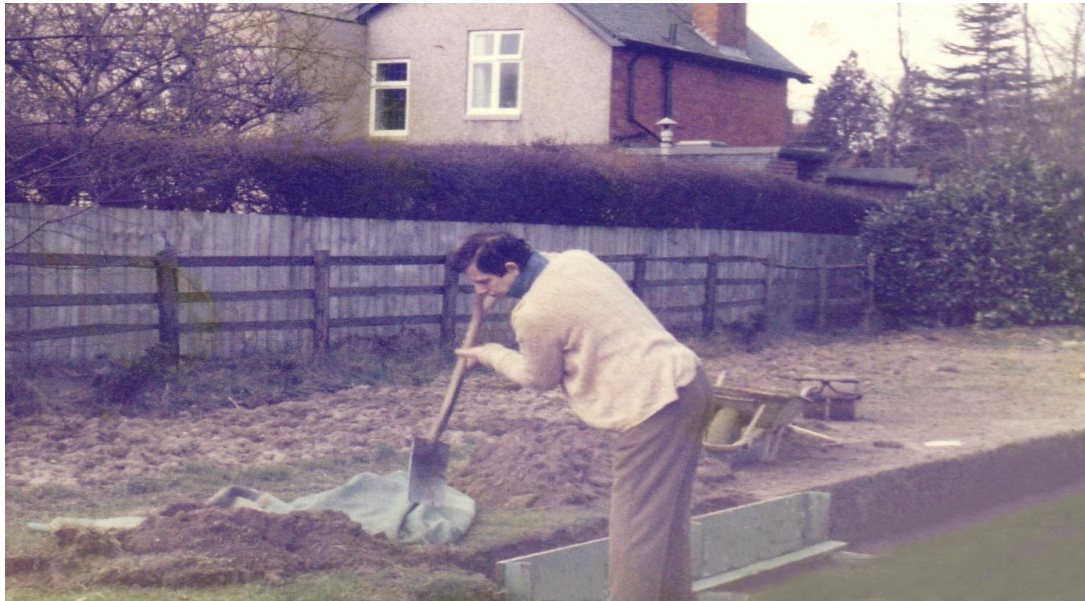
Construction of the bank-sides by the Secretary in October 1977 and completed in April 1979.
